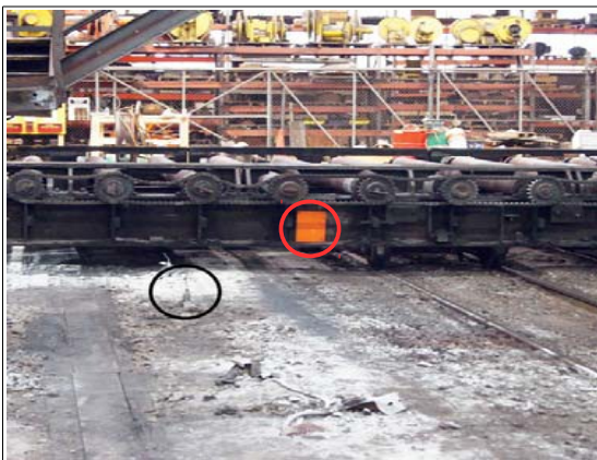
Pic 1: Mounted Target plate on transfer car
